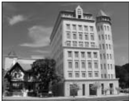
The top floor of the 83,000-square-foot office tower will house the Texas Center for the next ten years. Meeting space will allow the Texas Center to hold judicial conferences on-site.
